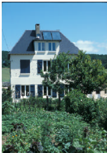
Chauffe-eau solaire, Fry.
